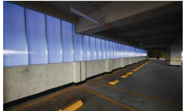
Car parking structures
